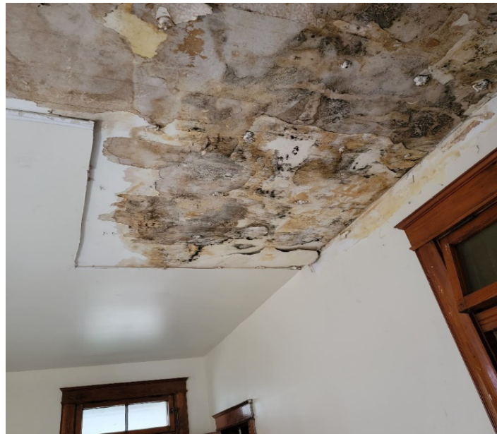
Figure 1. Moldy ceiling in one of the houses that the patient inspected.
